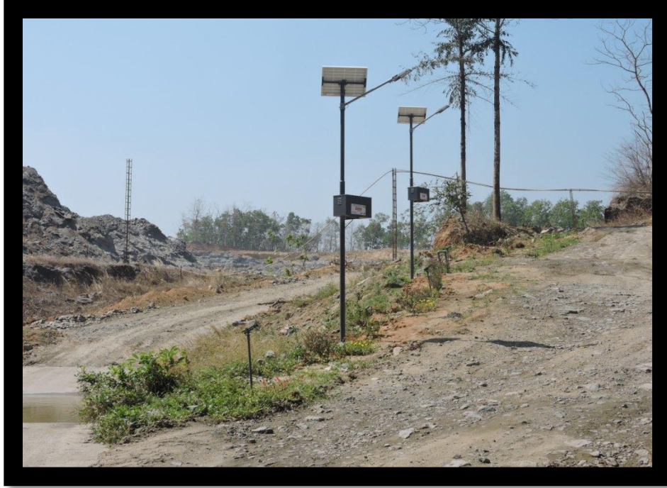
Solar light in the project site Plate No 4
