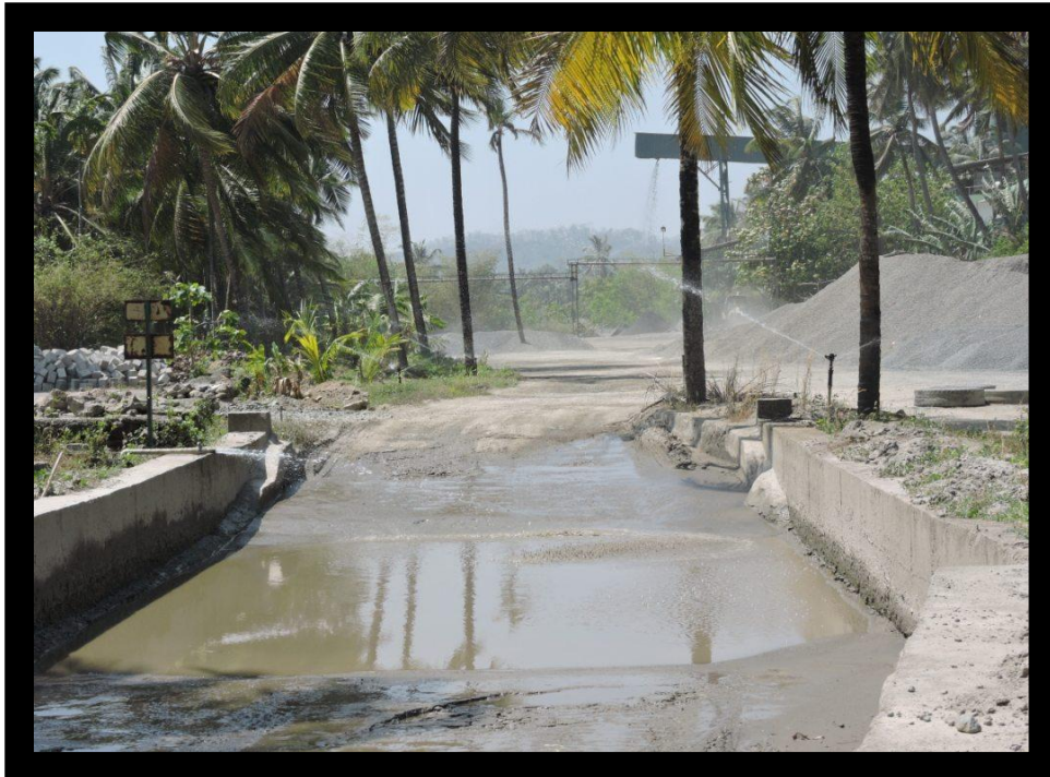
Sprinkler installed in project site
