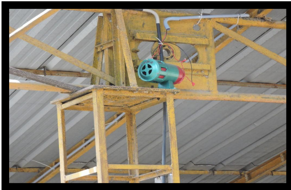
Warning alarm installed in the project site
