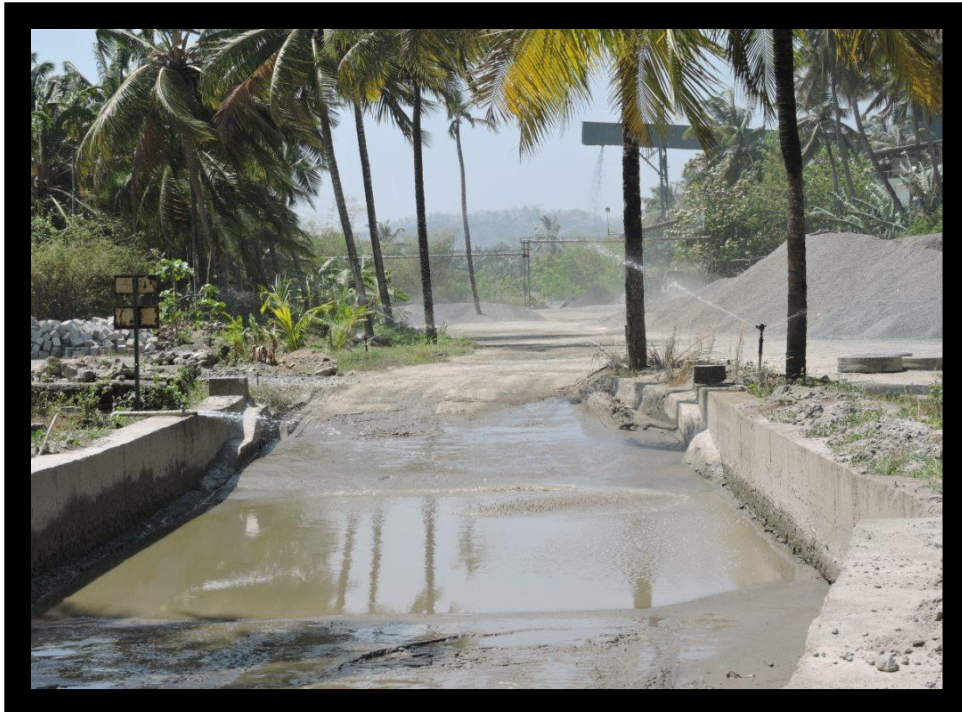
Sprinkler installed in project site
