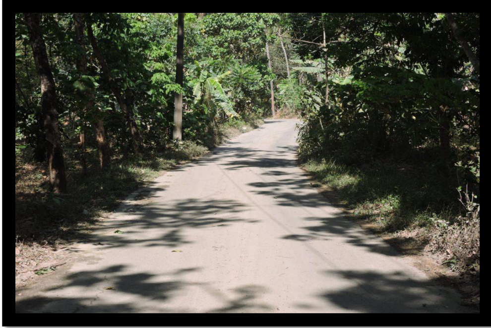
Tarred access road to the quarry site
