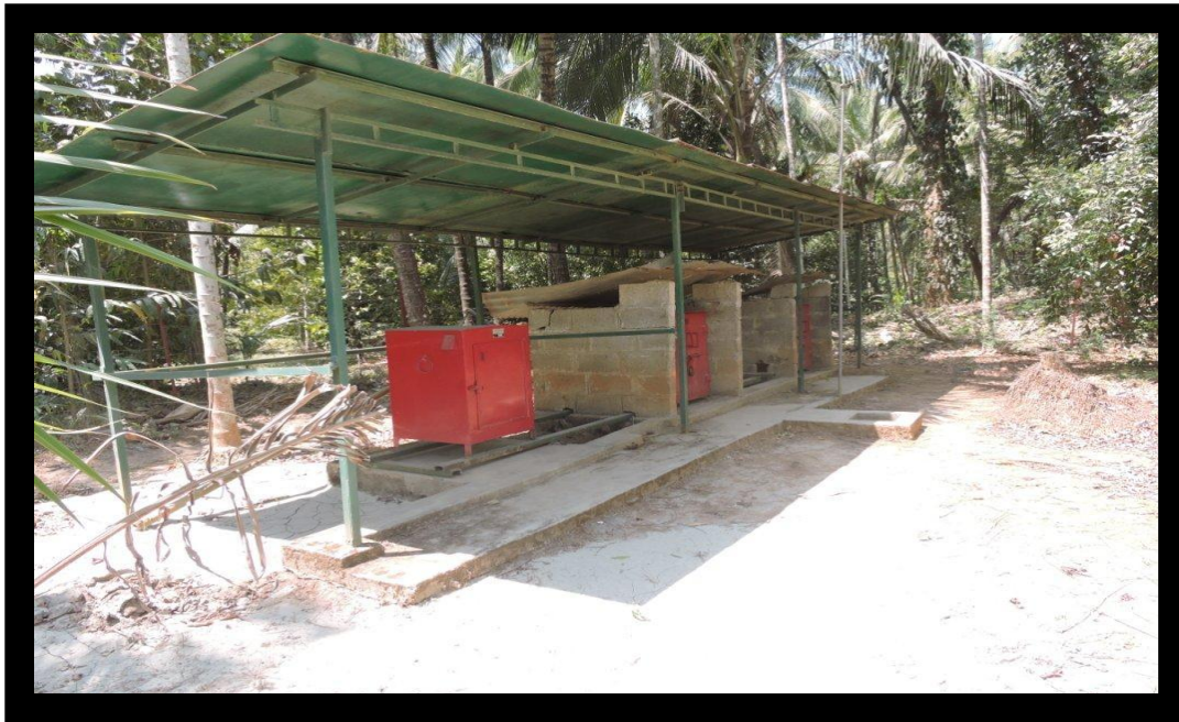
Magazines at isolated place in the project site
