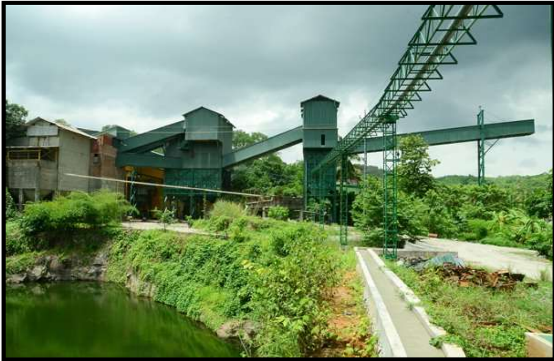
Crusher working in the project site
