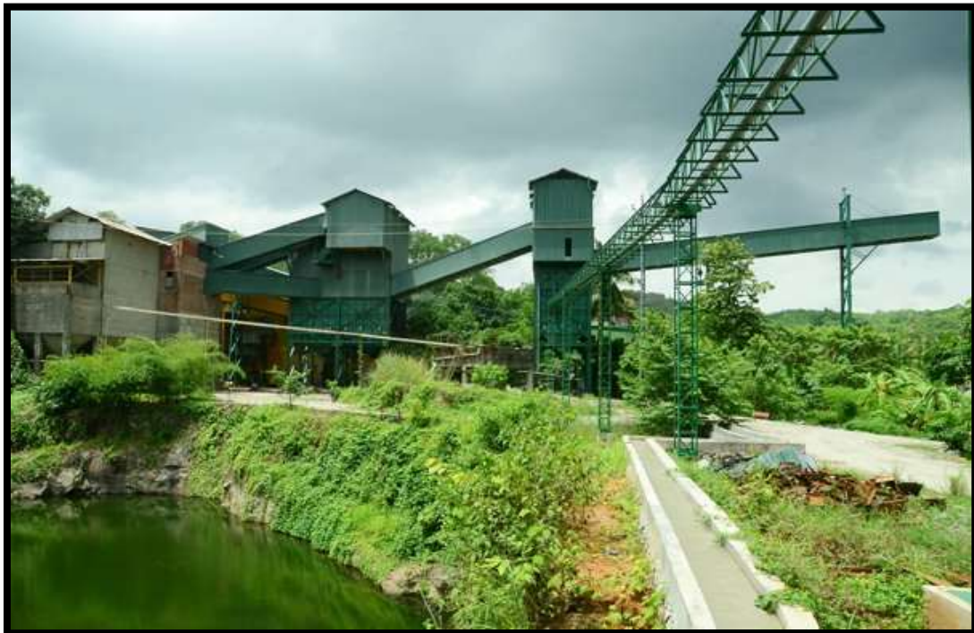
Crusher working in the project site
